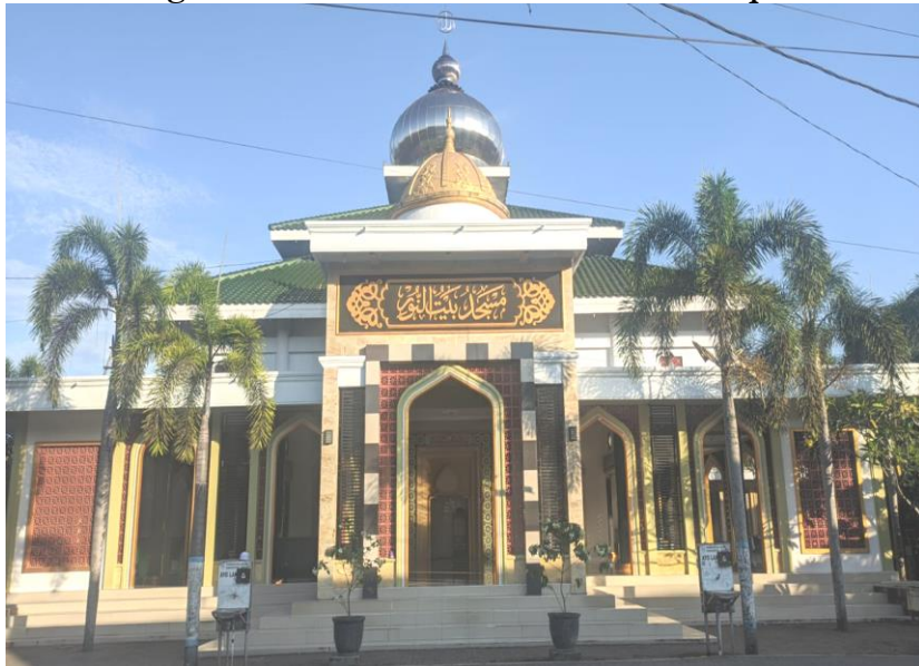
Figure 1. Front View of Baitun Nur Mosque
