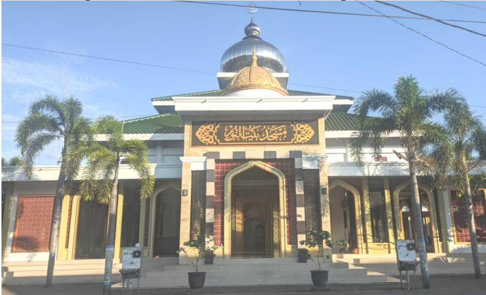
Figure 1. Front View of Baitun Nur Mosque
